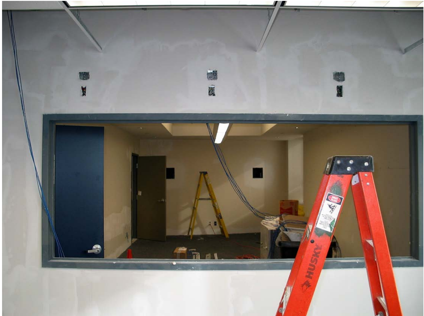
Market Research Center Construction of One-Way Observation Window
